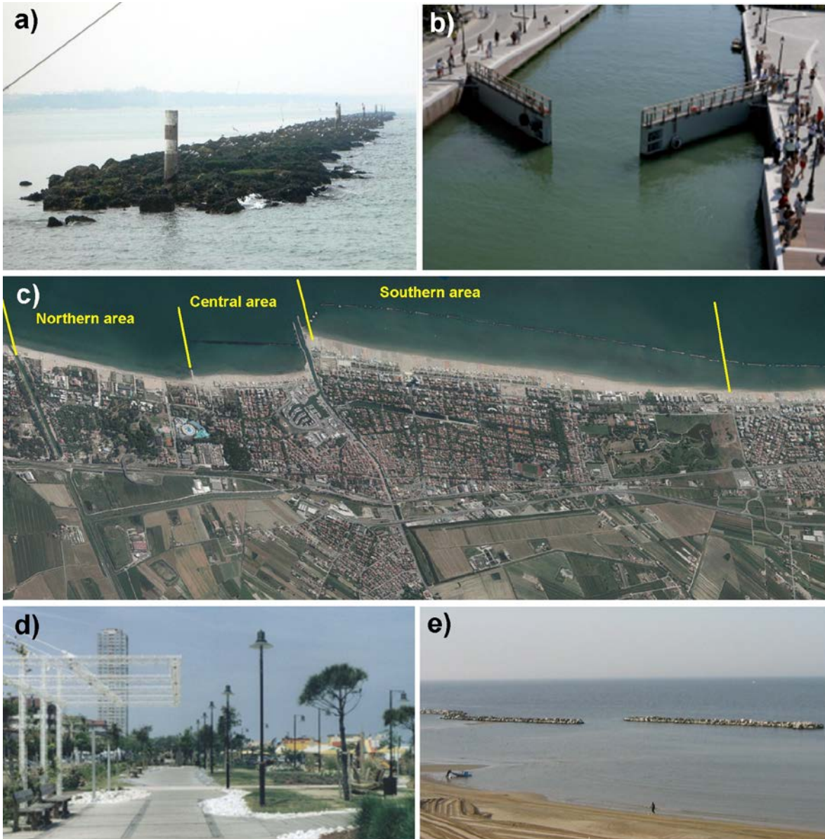
Figure 8.2. Aerial view of Cesenatico, subdivided into the areas recalled in the text, and pictures of the existing management a) semi-submerged barrier; b) sea gates at the Canal Harbour entrance; c) the “Gardens”; d) emerged barriers.
