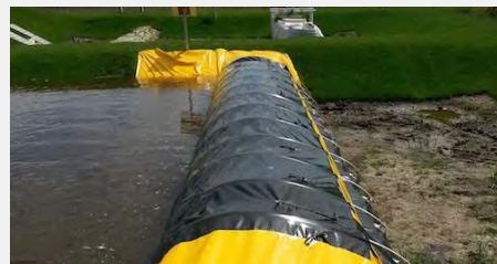
Figure 1 Schematic cross section of a Temporary Flood Barrier (left) and an example TFB (right) (source: www.tubebARRIER.com )
